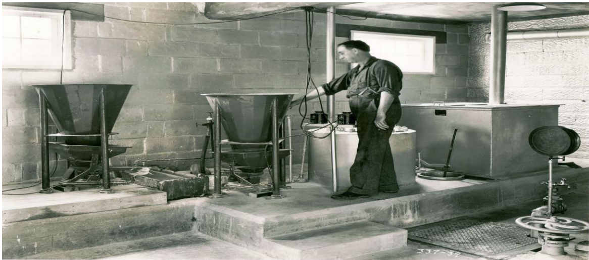
1939 Caldwell Water Works Lime Feeders
