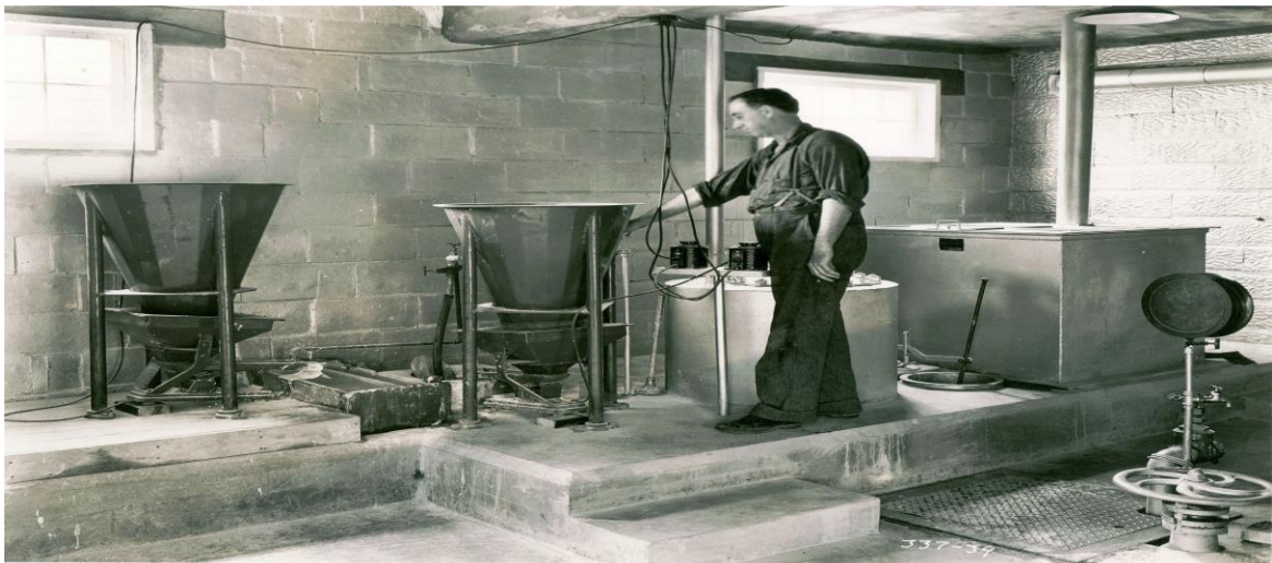
1939 Caldwell Water Works Lime Feeders
